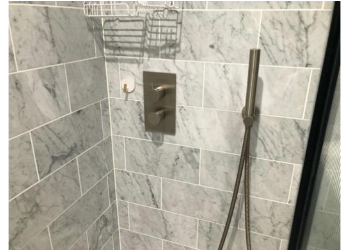
Condition of walk-in shower 2
