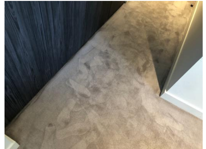
Condition of carpet 7
