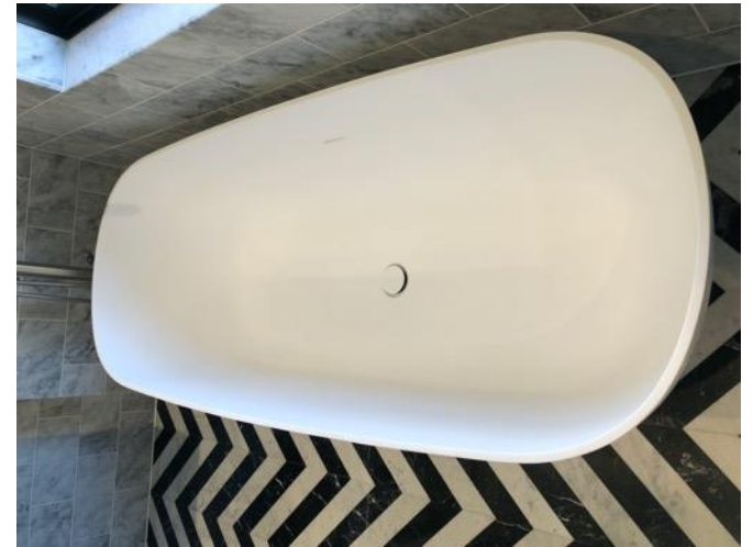
Condition of bathtub
