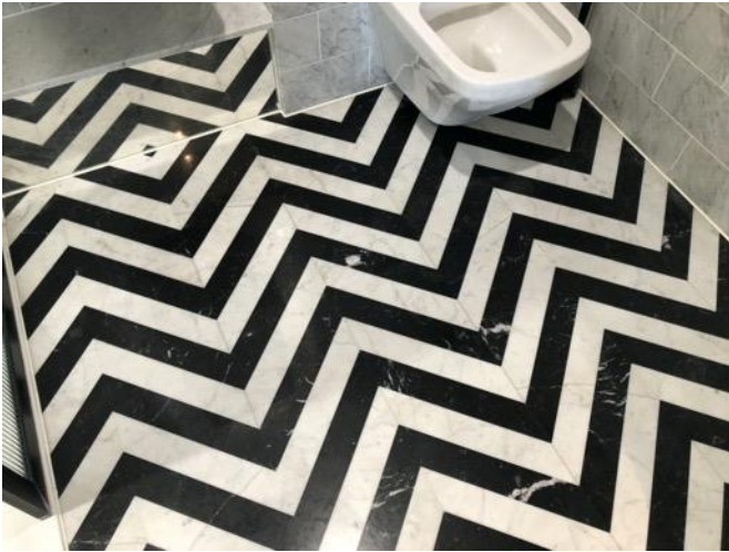
Condition of floor 1
