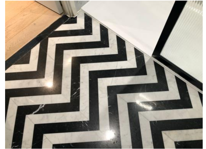
Condition of floor 3
