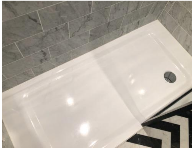
Condition of walk-in shower 1
