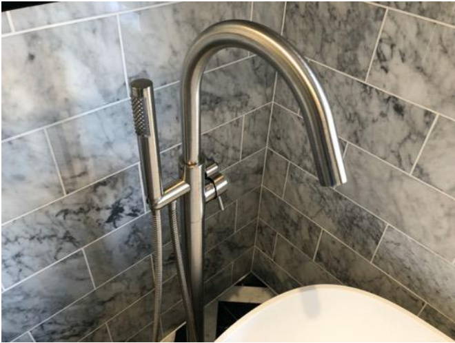
Condition of bath fittings
