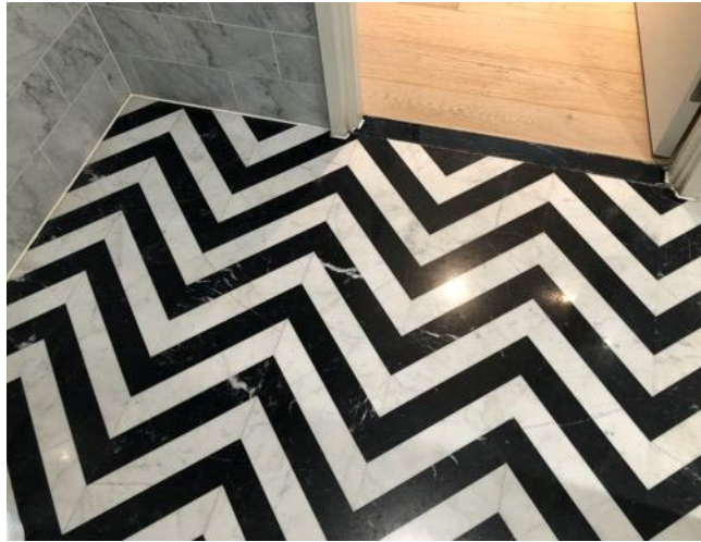
Condition of floor 2
