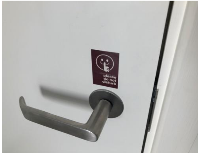
Sticker to exterior door (to reception)
