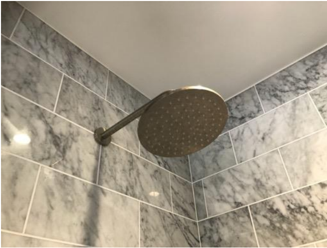
Condition of shower area 3
