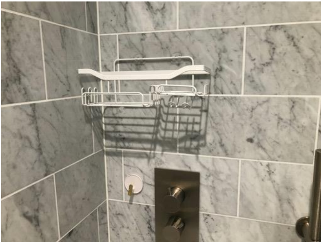
Condition of walk-in shower 3
