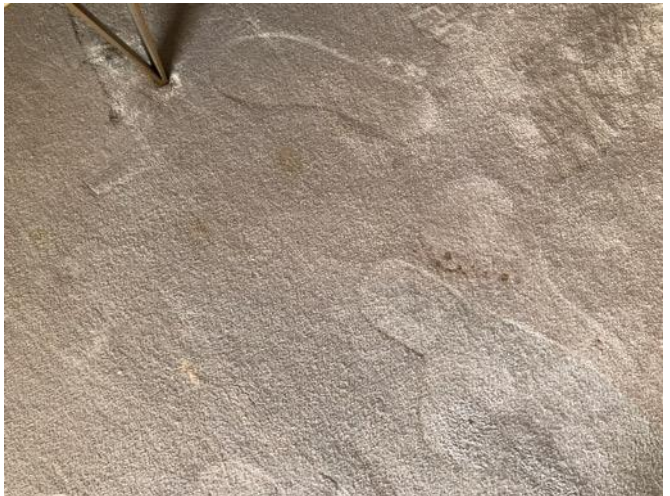
Brown staining to carpet around lhs bedside table 3
