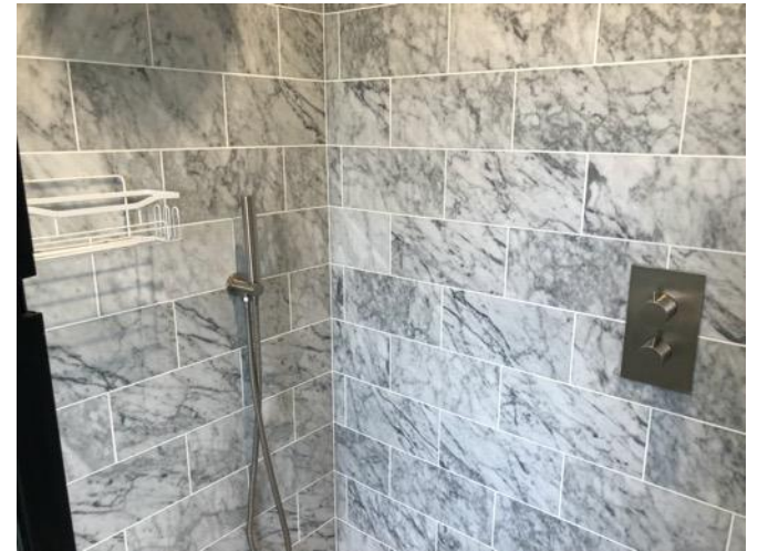
Condition of shower area 2
