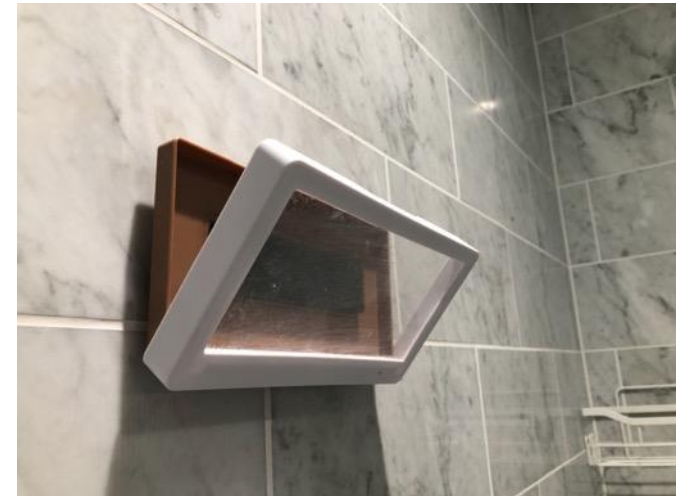
Condition of walk-in shower 5
