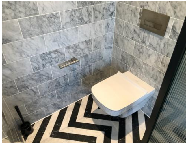
Condition of toilet area
