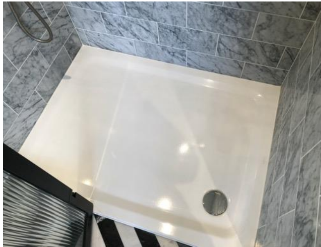
Condition of shower area 1
