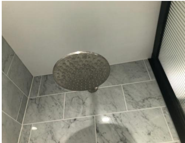
Condition of walk-in shower 4
